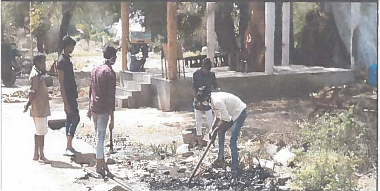
Volunteer cleaning the drainages at Nakkapeta Village
