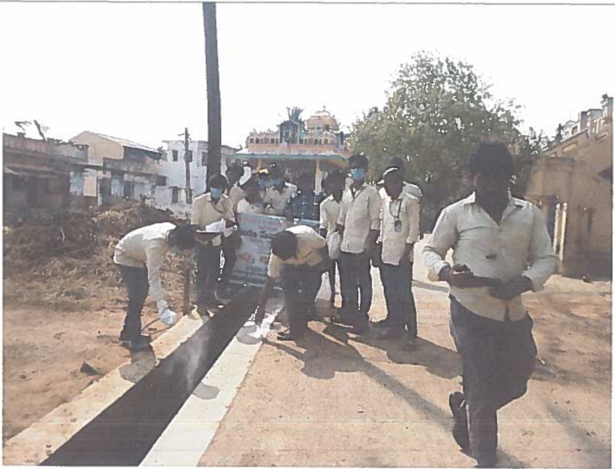
Volunteers chlorinating the drainages
