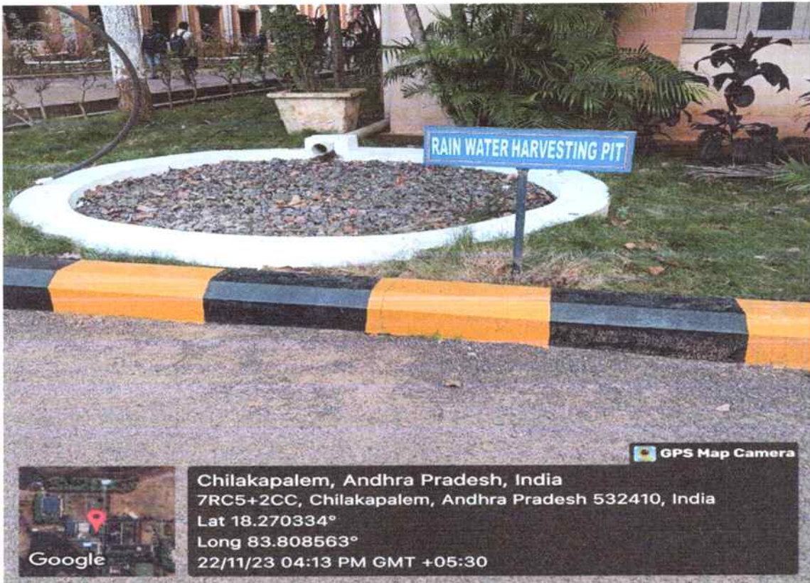
RAIN WATER HARVESTING PIT
