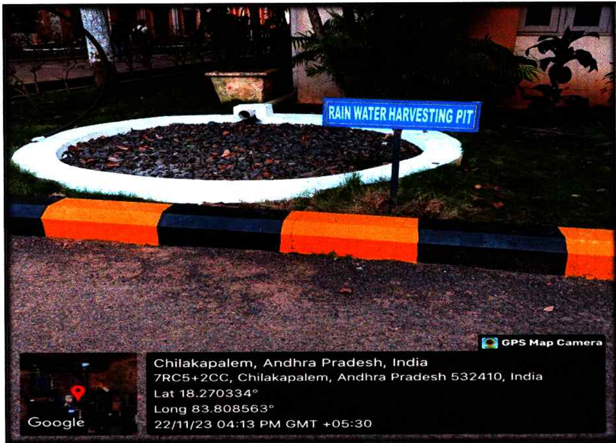
Rainwater Harvesting Pits in the College
