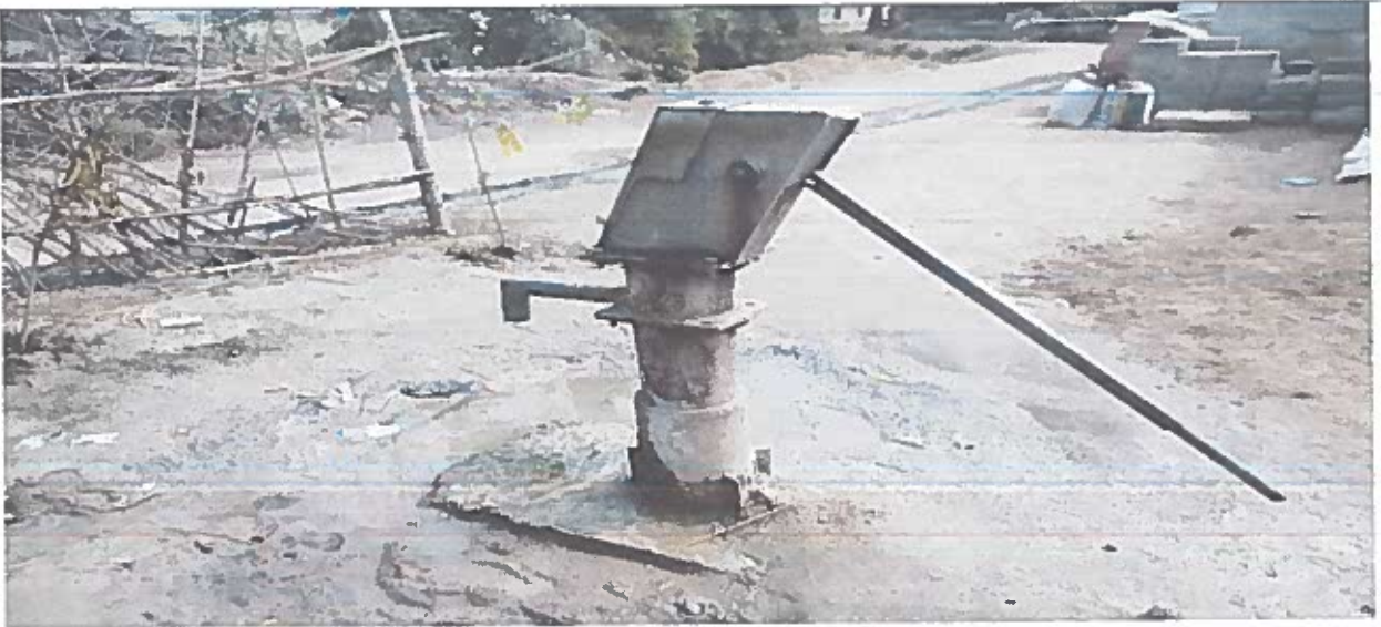
School handpump Before construction of platform
