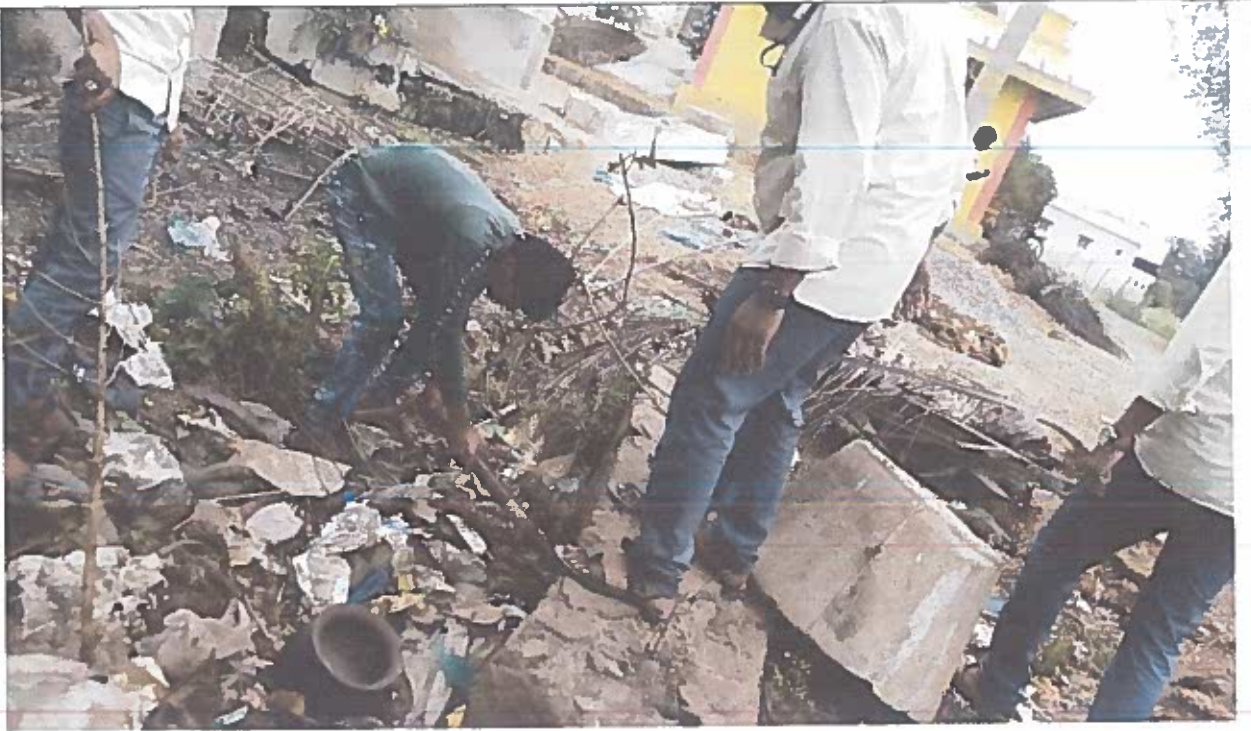
Drainages Before cleaning
