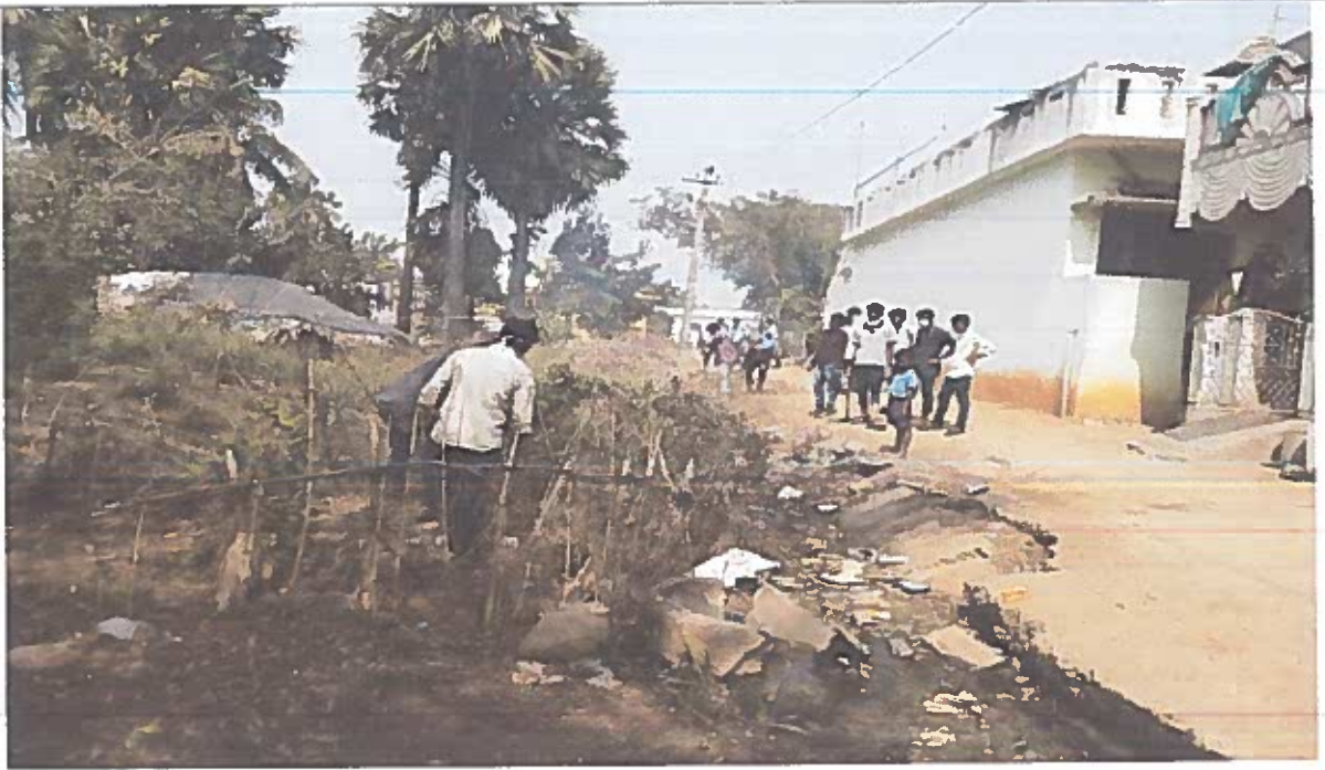
Drainages Before cleaning
