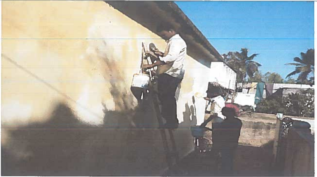
Volunteers Painting the school building
