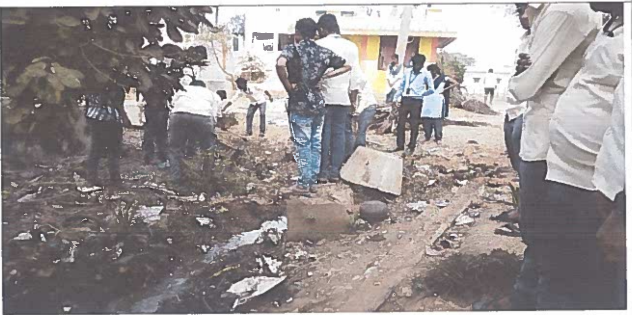
Drainages after cleaning
