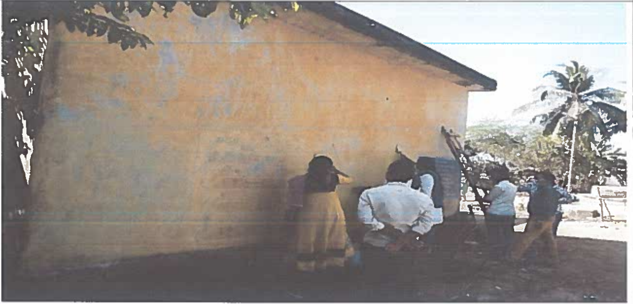
School Building Before Painting
